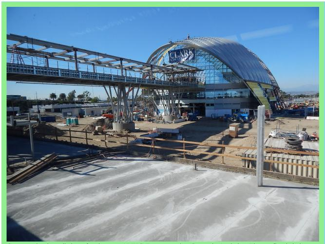
Construction is well along for the new ARTIC Transportation Center in Anaheim. The roofing is being installed and the new platforms are being built and extended to connect with the existing ones at Anaheim. Photo by Noel T. Braymer
