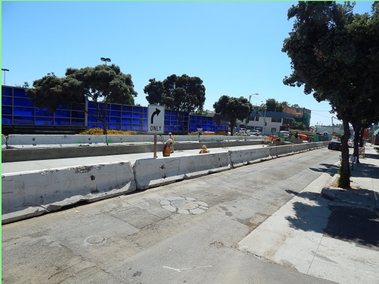
A photo this September of the work on Colorado Blvd in Santa Monica for the extension of the Expo Line to downtown Santa Monica. This is the median for the Expo Line's tracks in downtown Santa Monica near the terminus now under construction. Photo by Noel T. Braymer
