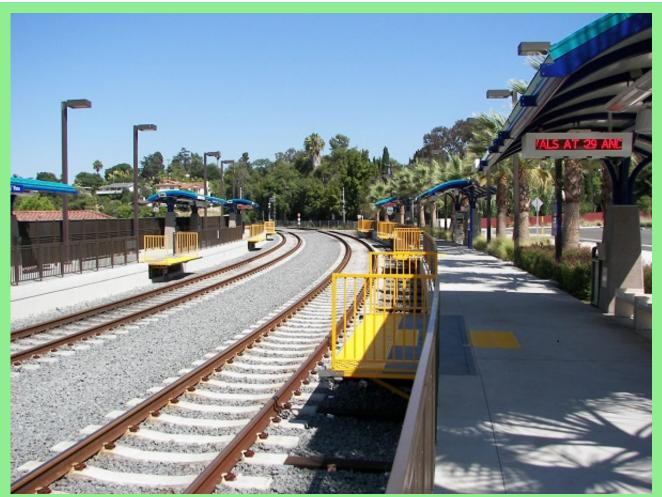
This is the Civic Center Drive Sprinter Station in Vista. With the use of drawbridges at the platforms it is possible to have level platform loading without building separate tracks for other trains. The drawbridges are raised at night so freight trains can use the tracks. With drawbridges it would be possible to have both high level and low level platforms at the same track. Photo by Noel T. Braymer
