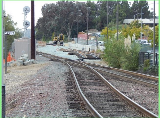
This is the start of a new mile segment of double track just north of the Sorrento Valley Coaster station which will be connected to the rail line between October 25-26. Photo by Noel T. Braymer
