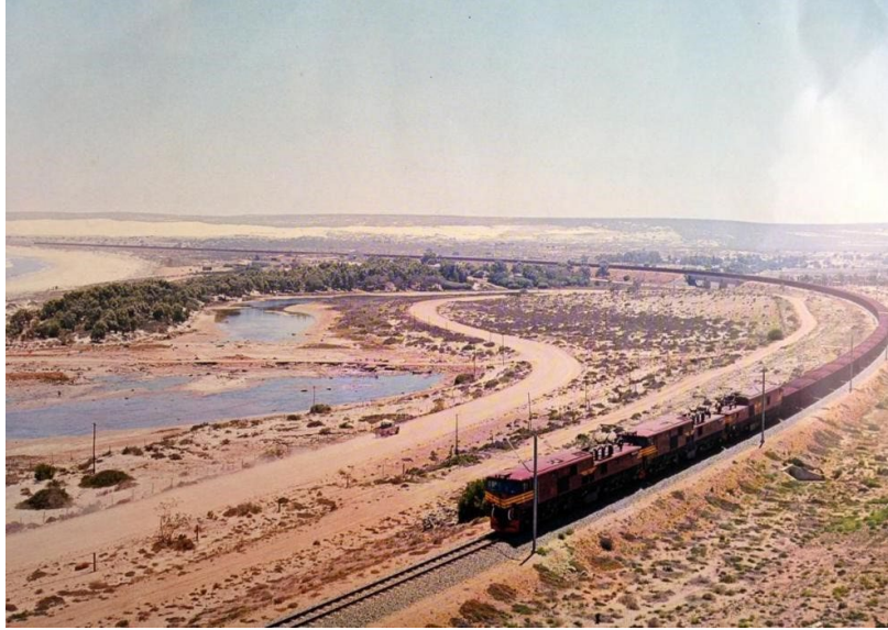
535-mile Sishen–Saldanha OREX line, South Africa: 40,000 ore trains in continuous operation under 50 kV catenary since 1976 (Photo: Peter Ball )
