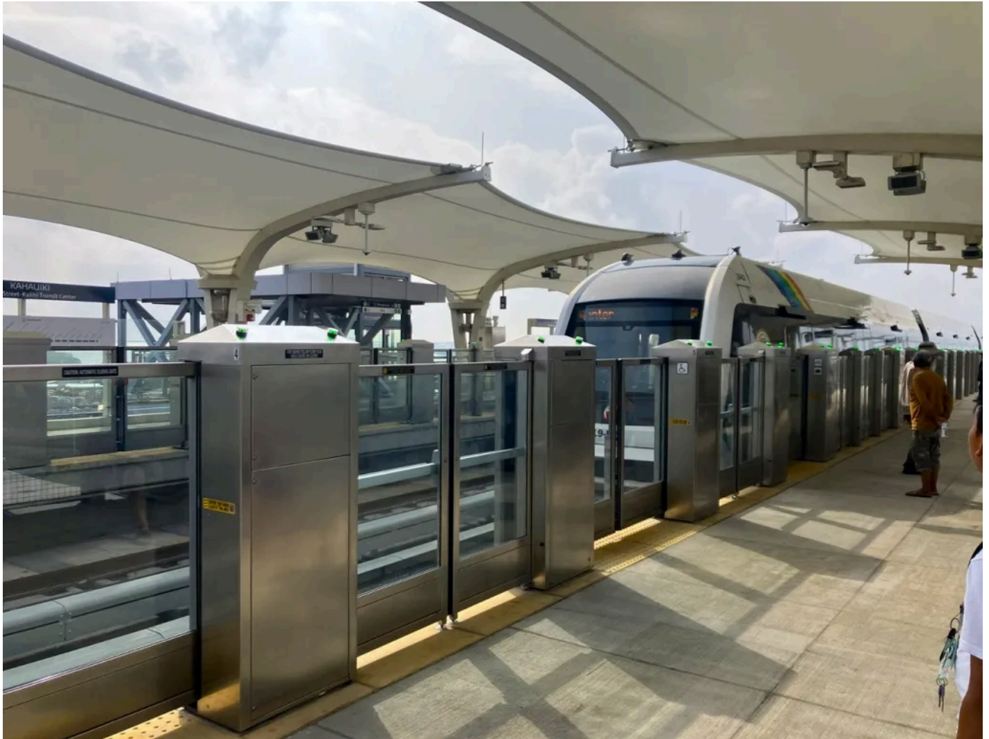
Platform screen doors (PSD) are at all Skyline stations, as seen here at the Kahauiki (Kalihi Transit Center) station, the current eastern terminus of the line.
